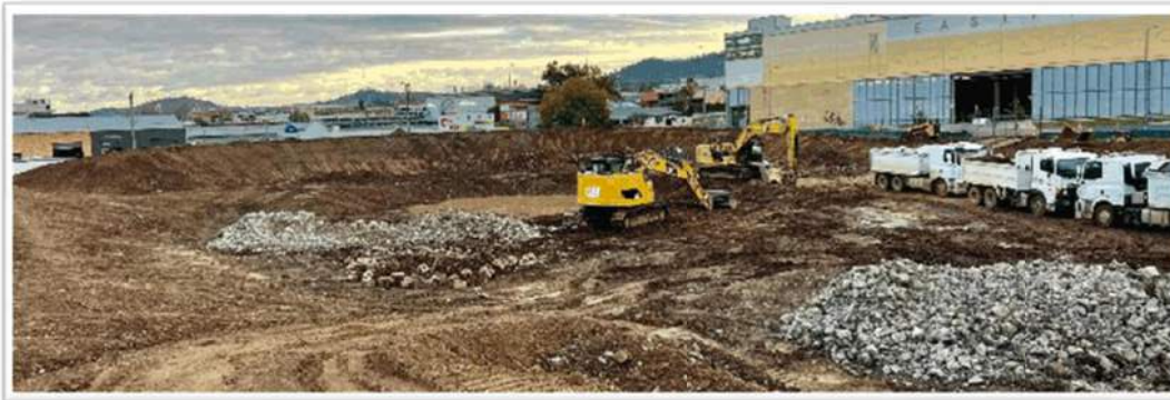
Council repurposed 1600 tonnes of concrete removed from the former velodrome site into road base material; diverting it from landfill.
